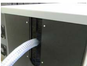
Pipe and cable are going through a polypropylene brush
